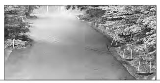
Photograph of the end of Lake Avenue in Georges Mills. This section of road was ground, regraded such that stormwater flowed away from abutting properties and Lake Sunapee, and into new paved swales and a cast-in-place catch basin at the low point of the road for improved stormwater treatment.
