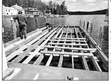
Photograph of the Harbor Dock Floor Joist **Project:** May 2021, In discovered that many of the floor joists under the decking of the north dock in the Harbor were rotting, and that two of the crib logs under the floor joist support structure were also rotten and causing sections of the dock to fall into the surface ofthe lake. Buildings & Grounds Department replace the floor joist rotten and crib logs
