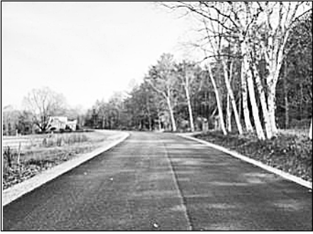
Stagecoach Road at top of hill looking east with rehabilitated drainage components, embankment improvements, 2" of new asphalt base course paving and new shoulder stone.
