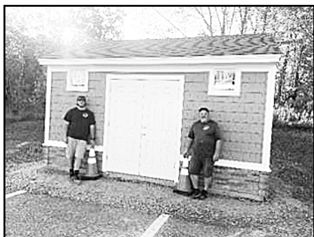
We love our new shed! Thanks to the foundation for sponsoring this project and to Craig and Darren for their terrific work building it.
