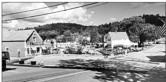
Photograph of the Main Street & Garnet Street Intersection Improvements Project. This project was originally designed, permitted, and bid out to local contractors in 2020 for construction in 2021. Early in 2022, the Town Manager and Highway Director worked with local citizens to establish a construction alternative (i.e. pavement markings) that allowed us to study two intersection realignment configuration options, and that also supports existing winter maintenance activities for this location.
