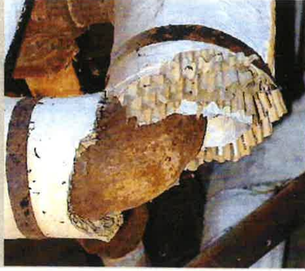
Damaged asbestos pipe insulation.
