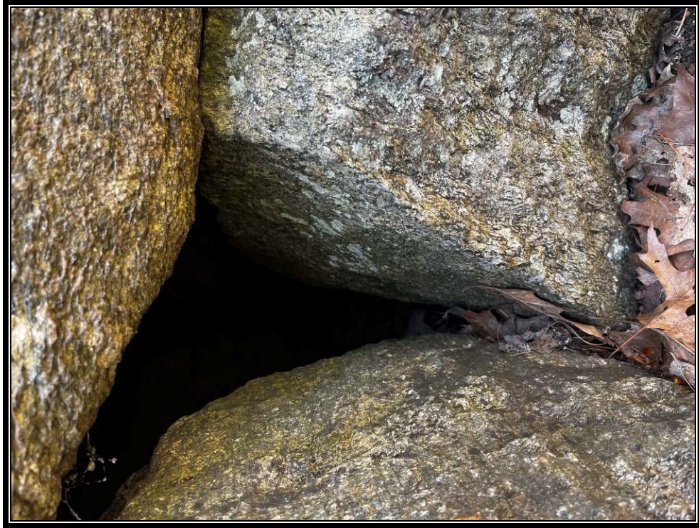
Photo 7: Large voids in the upstream wingwall.
