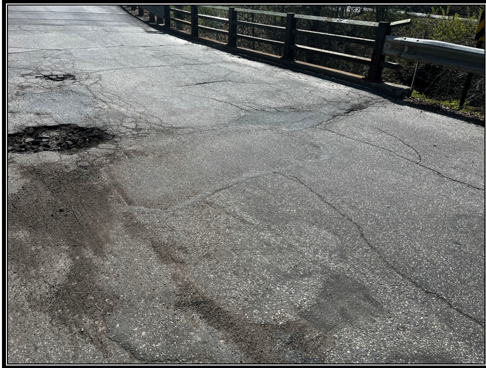
Photo 9: Large pothole reportedly patched last year.
