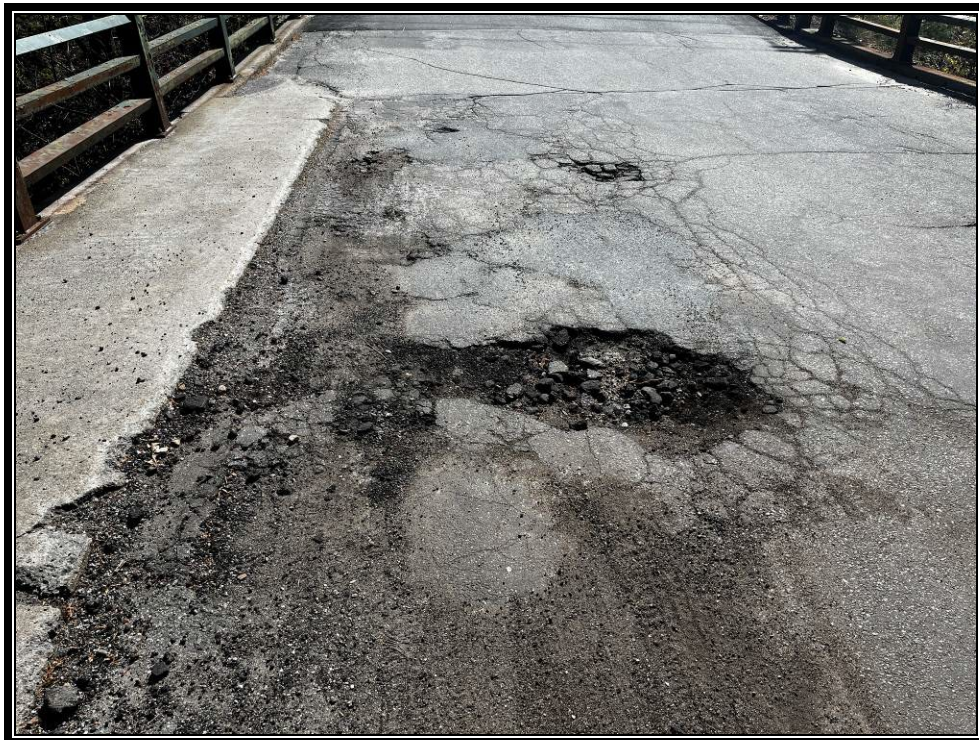
Photo 10: New pothole measured approximately 5 inches deep.
