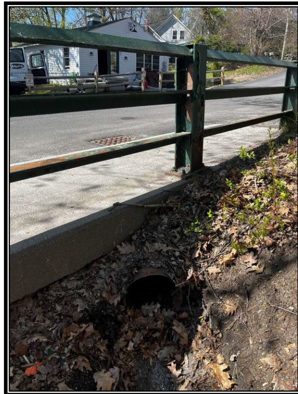
Photo 4: The upper catch basin outlet.
