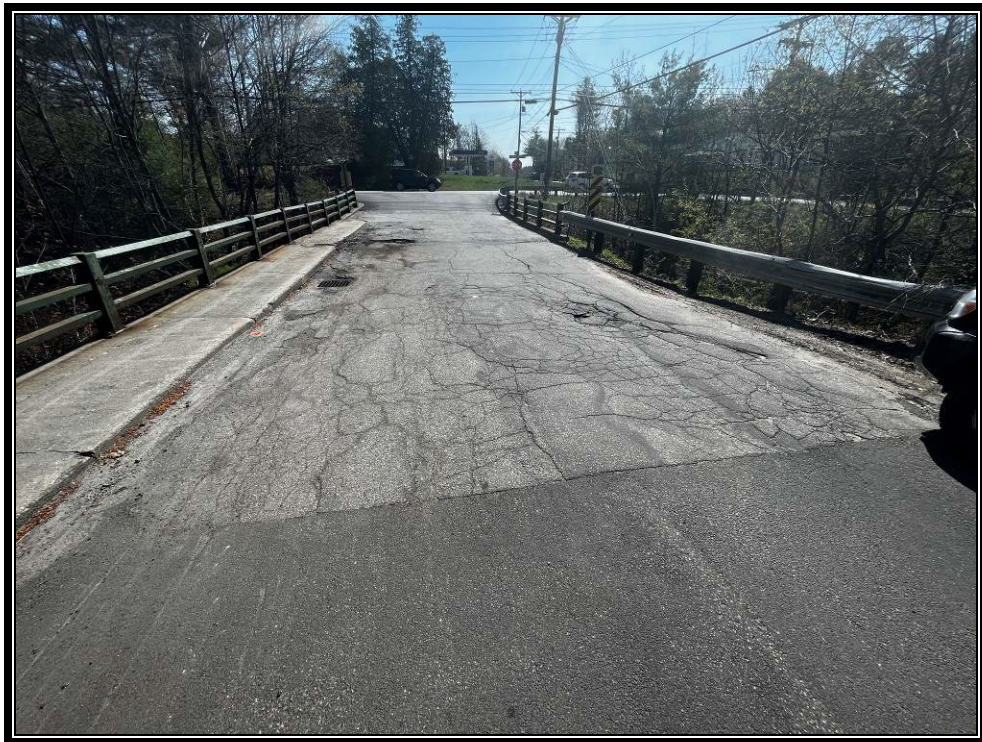
Photo 8: The pavement on the bridge in poor condition.
