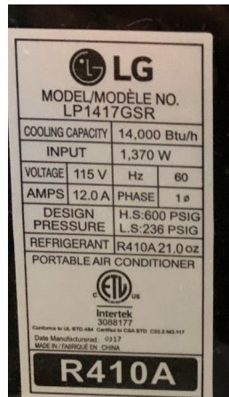
LG 14,000 Btu/hr floor standing, window vented AC unit serving second floor
