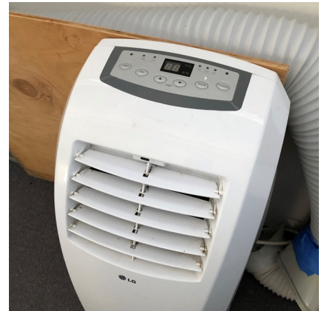
LG 14,000 Btu/hr floor standing, window vented AC unit serving second floor
