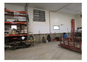
A large central exhaust fan is turned on manually as needed, drawing outside air through two louvred, screened openings along the same south facing wall.
