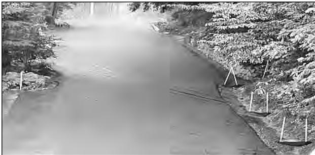
Photograph of the end of Lake Avenue in Georges Mills. This section of road was ground, regraded such that stormwater flowed away from abutting properties and Lake Sunapee, and into new paved swales and a cast-in-place catch basin at the low point of the road for improved stormwater treatment.
