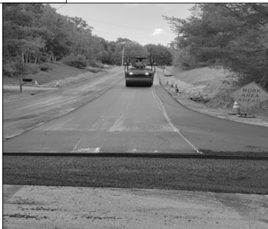
Photograph of the resurfacing of Dowd Lane with the rehabilitated stone-lined drainage ditches on both side of the road.
