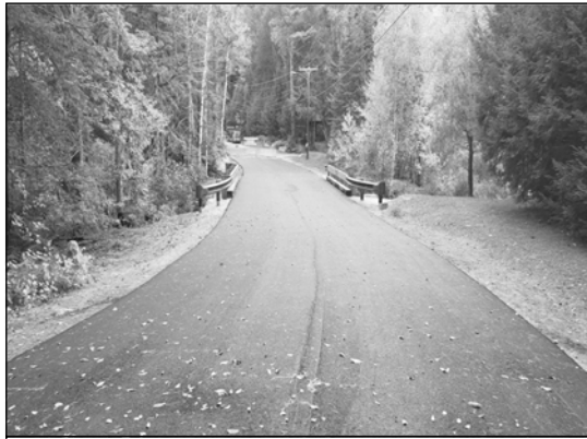
Photograph of Jobs Creek Road Bridge over Jobs Creek replaced with a laminated wood beam and laminated wood deck bridge, paved over and with new wood and corr-10 steel guardrails.
