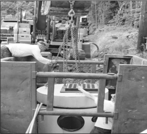
Photograph of the installation of a pre-cast concrete catch basin in preparation for the reconstruction of Stagecoach Road.
