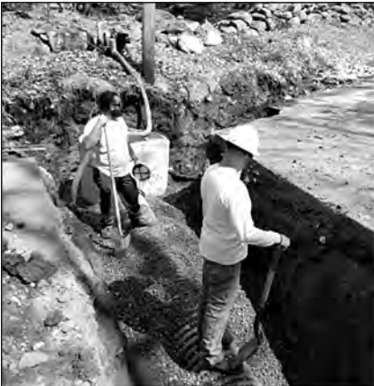
Photograph looking south to north across Perkins Pond Road of the installation of a pre-cast catch basin and a 15" HDPE cross-culvert pipe in preparation for the reconstruction of the paved section of Perkins Pond Road.
