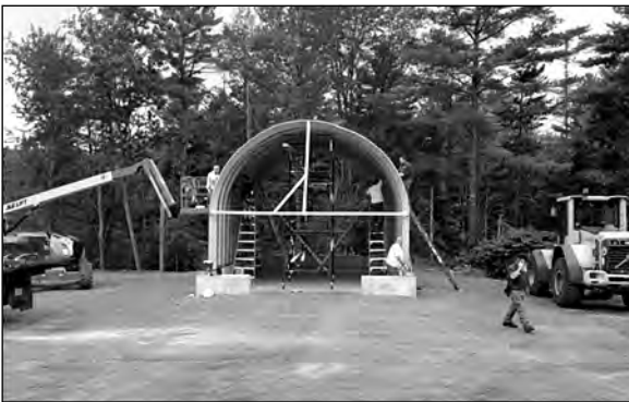
Photograph looking east to west at the front of the Quonset hut prior to the installation of the west end wall and the vinyl garage door.
