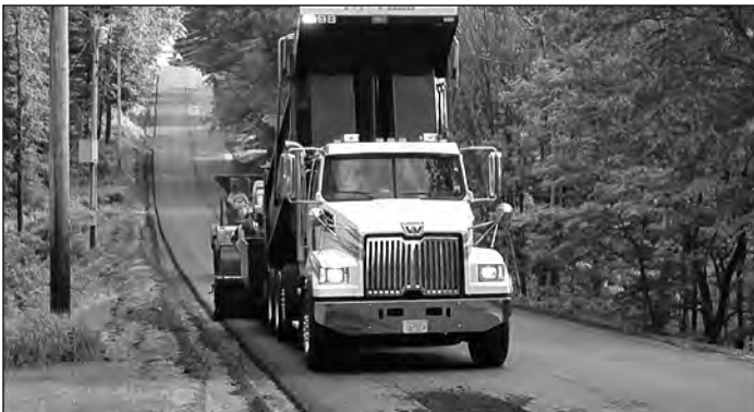
Photograph of North Road (near the cemetery) with the top course of pavement being installed on the roadway.
