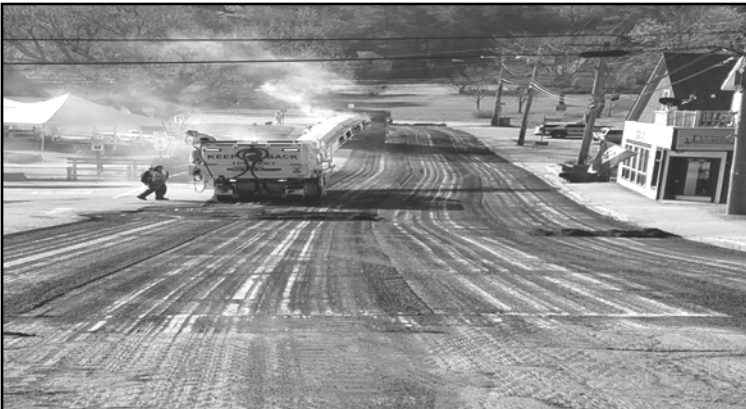
Photograph of Main Street coming into the Harbor being cold planed in preparation for re-surfacing.
