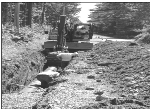
Photograph looking north to south along the east side of Ryder Corner Road of the installation of the 15" HDPE trunk line
